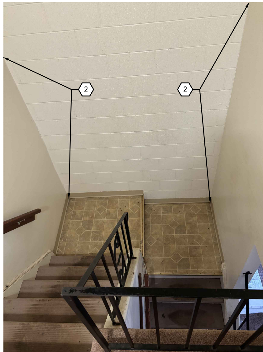
C VIEW OF TAN CAULK - STAIRWELL H100
